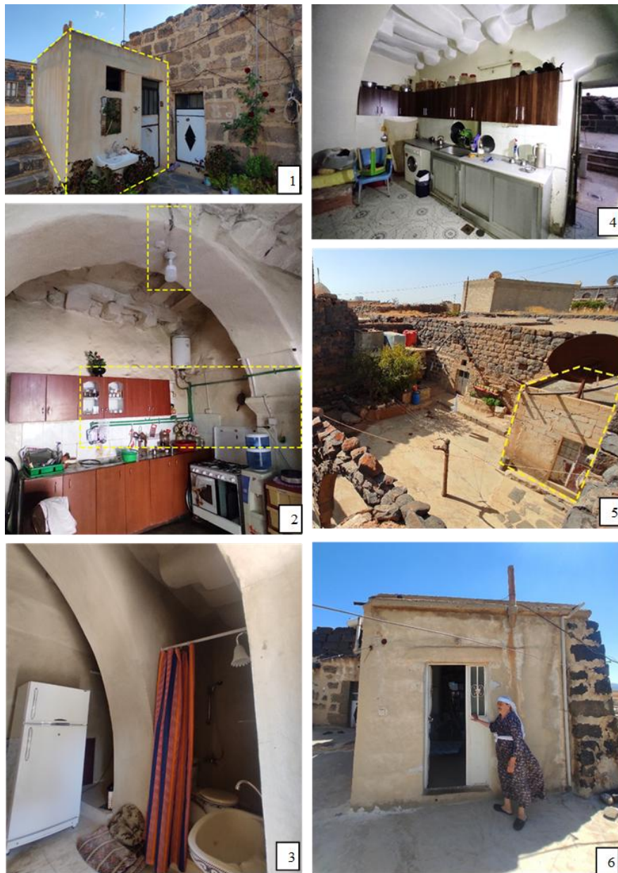
Fig. 12: Different ways of adding amenities (Kitchen and toilet): External concrete addition 1,5,6. Incorporating amenities within the structure 2,3,4.
