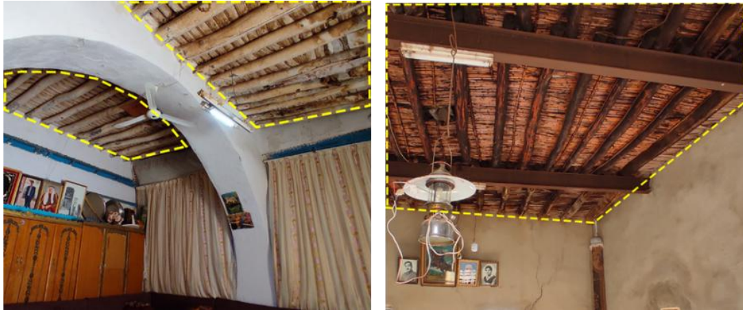
Fig. 6: Change in roof structure, using wooden beams and keeping the arch, replacing the arch with metal beams.
