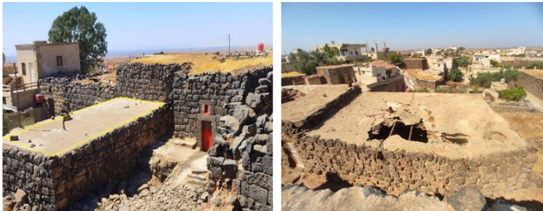
Fig. 5: Applying a concrete layer on top of the original roof layers. Shaqqa, Melah.
