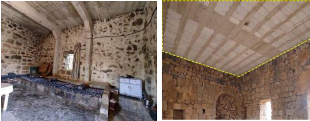
Fig. 7: Replacing the original roof structure with reinforced concrete. Qanawat.
