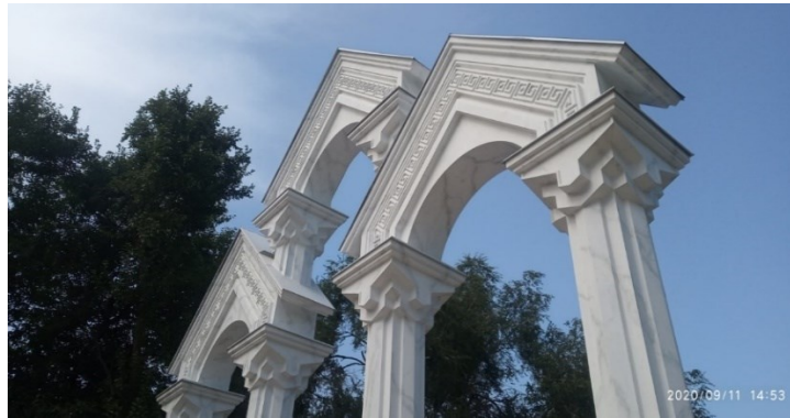
Fig. 7. Stellate trunk of the column, stalactite capital, and the arched roof with a moulding of Kazakh ornament
