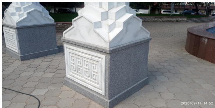
Fig. 6: Curbstone pedestal with a rosette of Kazakh figured ornaments and a stalagmite base of the column Source: prepared by the authors
