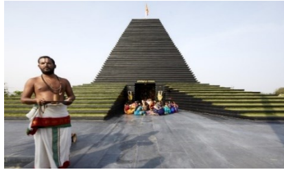
Fig. 26: Stepped platform with green cover providing a soothing environment
