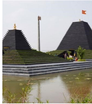
Fig. 25: Water bodies around temple structure giving cooling effect
