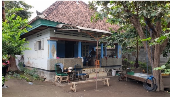
Fig. 3: Façade of the the old house Source: Authors, 2018
