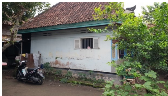
Fig. 7: Side view of the old house Source: Authors, 2018
