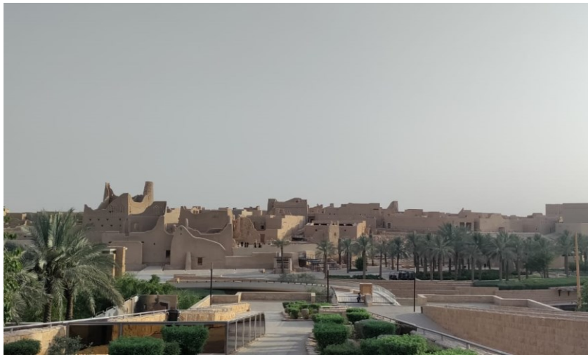
Fig. 6: Regenerated Al Diriyah prior to its public opening in August 2022. Source: Author
