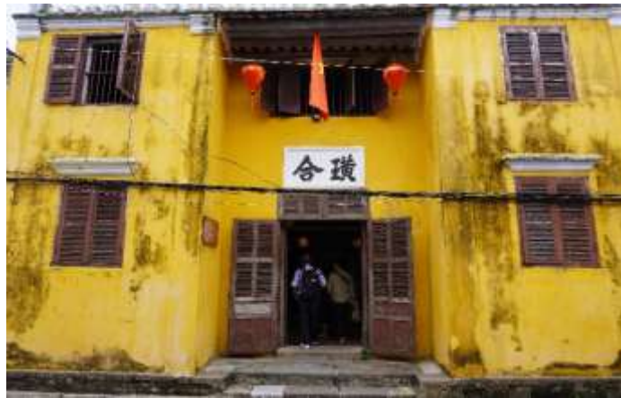
Fig. 1: The facade of Hoang Hiep ancient house.
