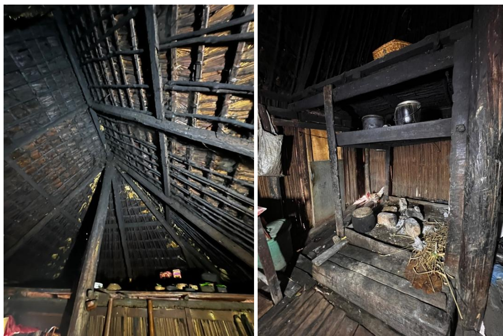
Fig. 4: Interior views of a traditional Kamanasa house (B2).
