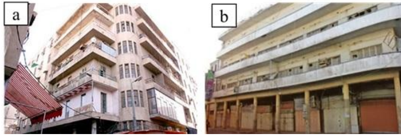
Fig. 2: (a) Damarchi building, (b) Sofair building. Source: Al-Sultani, 2014
