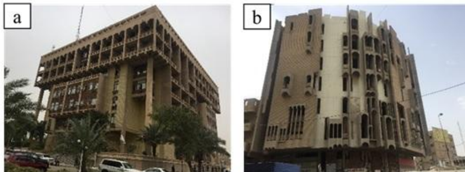
Fig. 10: Use of shanasheel, (a) Liquefied water building, (b) Industries union building.
