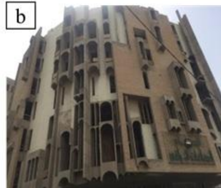
Fig. 3: (b) Industrial union building Source: Author
