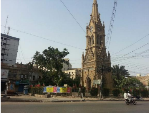
Fig. 9: Electrical Lines around the tower.
