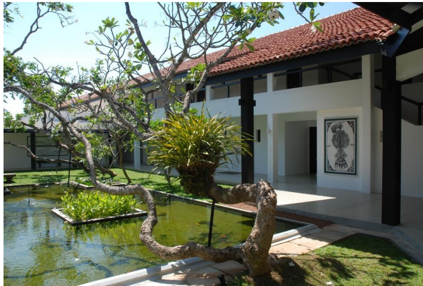
Fig. 3.3.2: Serendib Hotel, Bentota - View of the Entrance Court.
