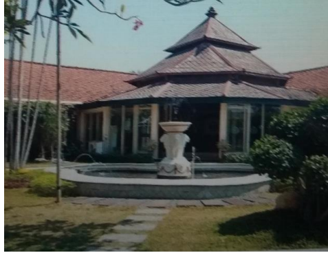
Fig. 5: The Shape of the Tajug Roof of the Pracimayasa Building at Mangkunegaran Temple Source: Author
